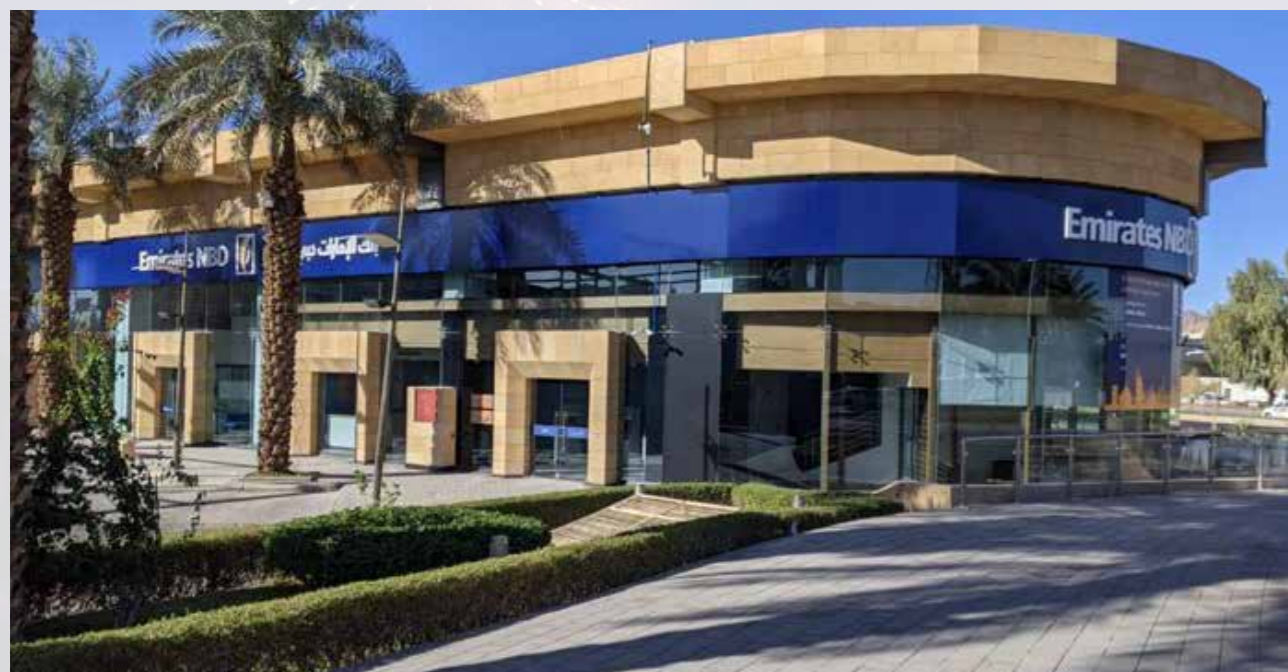
Emirates NBD expands its presence in KSA
