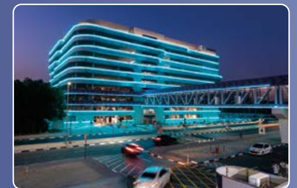
Emirates NBD is the first bank in the Middle East to receive Parksmart Gold certification for its Nad Al Sheba parking facility
