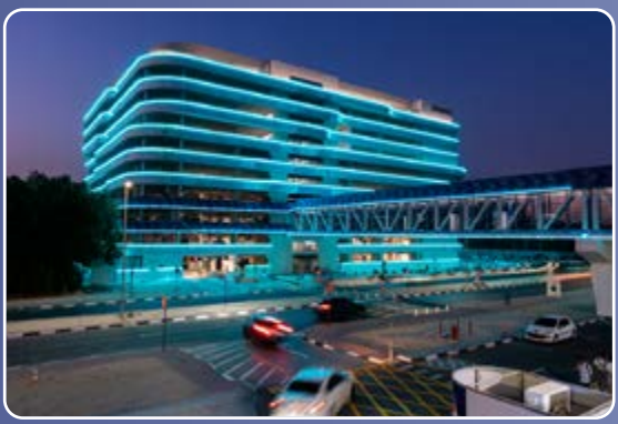
Emirates NBD is the first bank in the Middle East to receive Parksmart Gold certification for its Nad Al Sheba parking facility
